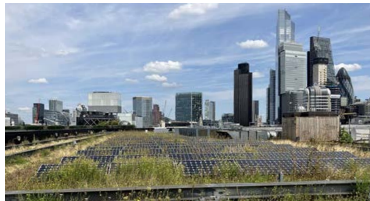
Image: Biosolar roof installation at Watermark Place Source: City of London Corporation
