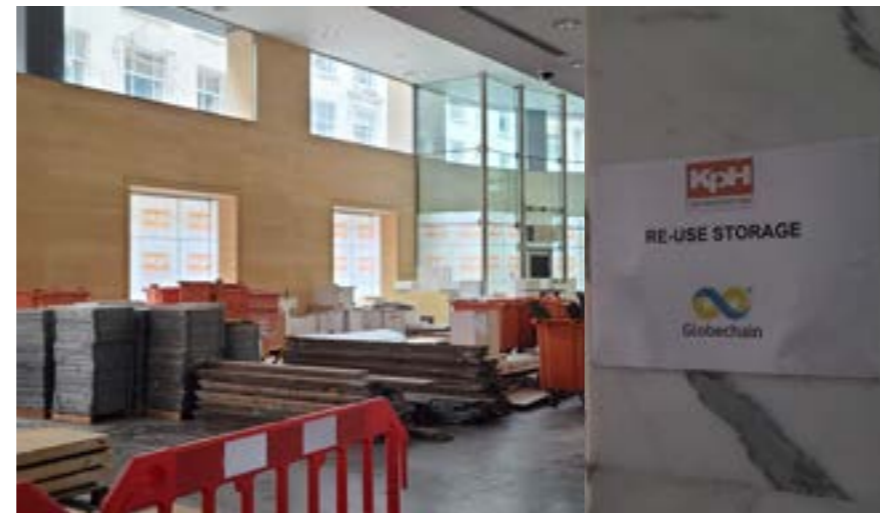
Images: Salvaged materials being processed on site at 75 London Wall Source: City of London Corporation
